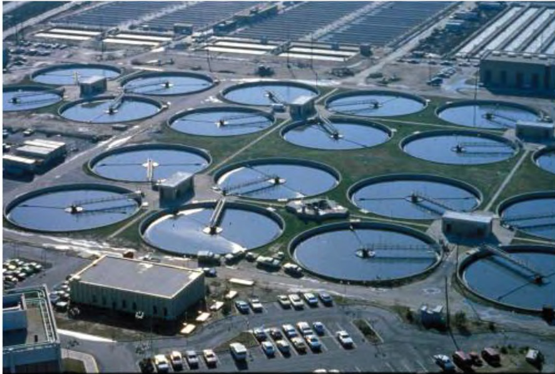
Figure 25.1 Sewage Treatment Plant (credit: "eutrophication&hypoxia"/flickr.com)
